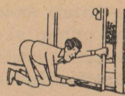
Weatherstrip all outside doors
