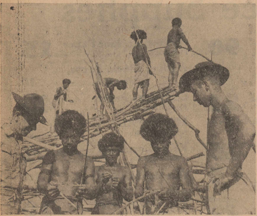
There is no timber in New Guinea, and so, when it comes to building, the American soldiers learn a trick or two from the natives near Port Moresby. Before the grass thatch is put on, the beams are securely tied with strips of bark which the natives are shown peeling. In the background the framework of one house is all but completed. Little forks that two of the natives wear in their hair are solely for pleasure—the pleasure of scratching.
