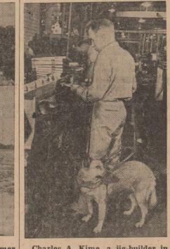
Charles A. Kime, a jig-builder in a Burbank, Calif., aviation plant, lost his sight in an accident. Now he is back at work in the same factory, and is pictured here installing rivet nuts for the de-icing boot on the leading edge of P-38 empennages.
