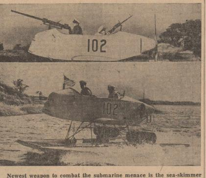
sub-chaser, which hops the waves at 50 miles per hour. It is armed with four depth charges, which can be replaced by torpedoes. Except for the engine and propeller, it is built entirely with non-strategic materialplywood plastic-and can be molded out by the thousands in a short time. As it is not driven by a water propeller it cannot be detected by submarines. Top photo shows the two-man crew at the guns. Bottom photo shows the sub-chaser skimming over the water.
