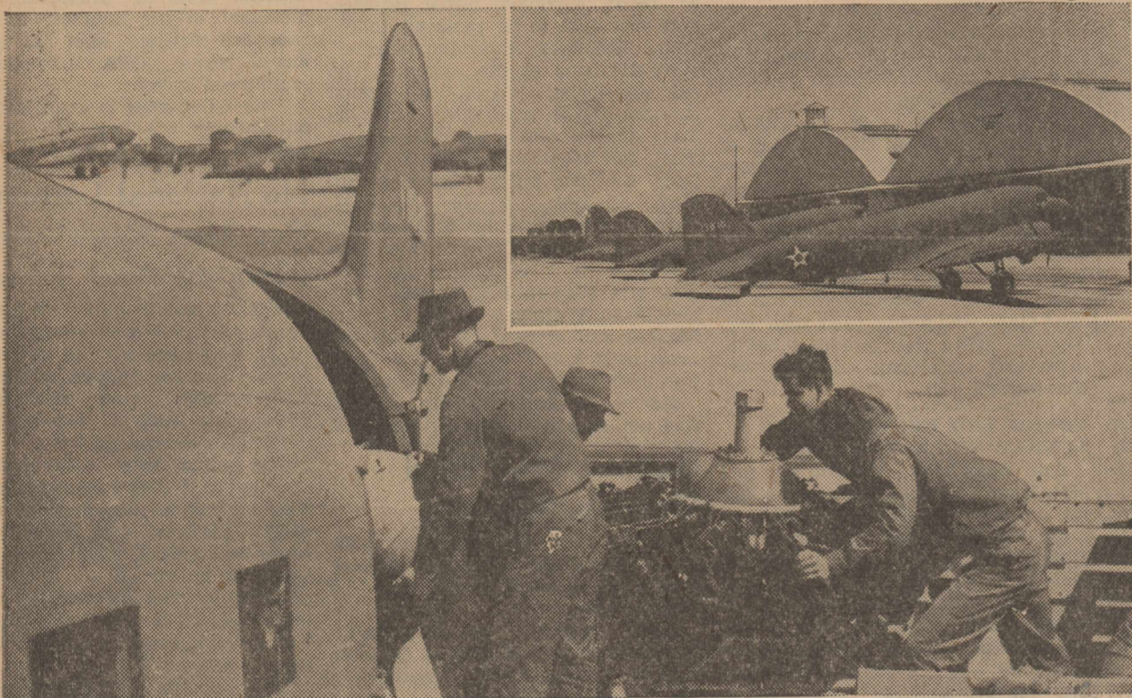
At an army air depot somewhere in the western part of the U. S., huge transport planes, "the flying box-cars" of the army air force, ship freight on wings to foreign battle fronts. At left the loading crew is transferring freight to waiting "flying box car." Inset: Poised for flight are these air freight planes, to any air field in case of an emergency call.
