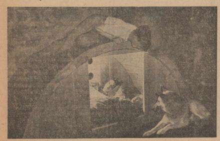
If the brick of this house comes tumbling down, the mother and two children inside this timber air raid shelter would be fairly safe. The heavy timber is easily put together with pegs, contains a double bed got drenched when his P-38 interand incendiary bomb fighting equipment. The family is bundled in for the night, with one son on top, looking on-and the dog looking in.
