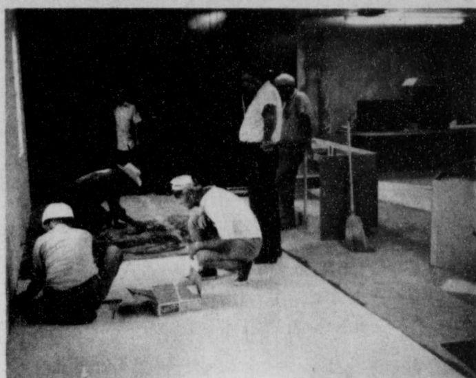
ROBY FIREHALL: Above is a picture of the newly re-modeled Fire Hall building in Roby. All the work was done by volunteer firemen to include completely re-doing the inside, installing a new ceiling air conditioning system, new rest rooms, and a new floor. The new building is going to be used as a meeting place for the firemen, a community building, and a site for family re-unions. Pictured are Kidd Waddell, Pete Driver, Ruben Rodriguez, Howard Fought, J. M. Whitfill and Wayne Pursley. Plans are to remodel the exterior in the near future.
