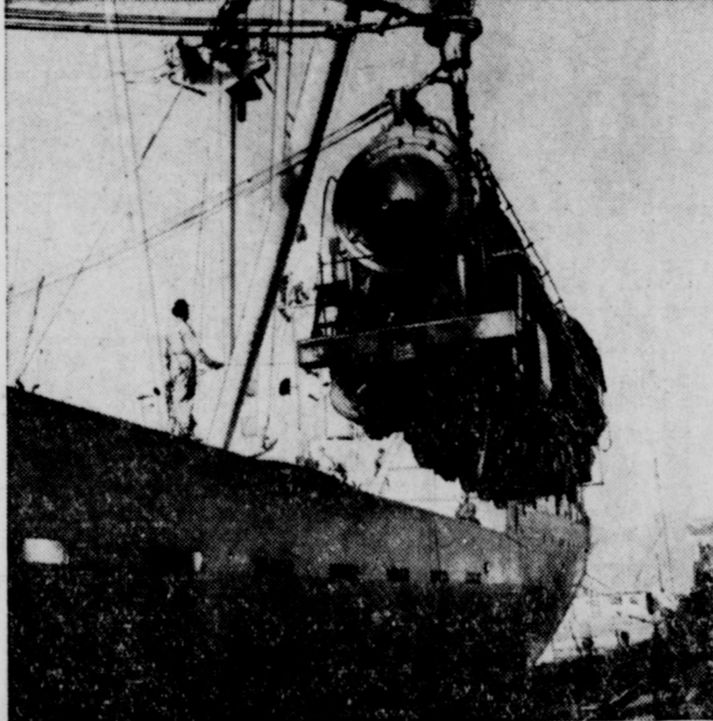
IRON HORSE FOR EUROPE . . . Crushed and broken Europe, more than two years after the war's end, still is striving to rebuild. With the aid of American equipment the iron continent is being reshaped. Here, a 115-ton engine is hoisted into the hold of the S. S. Beljeanne at the Erie railroad yards, Weehawken, N. J. The iron monster is part of a shipment of 29 rail locomotives being sent to Poland to restore that nation's war blasted rolling stock. One of the hardest hit of all European nations, postwar Poland found herself trying to reconstruct with her transportation system virtually in a state of total paralysis.
