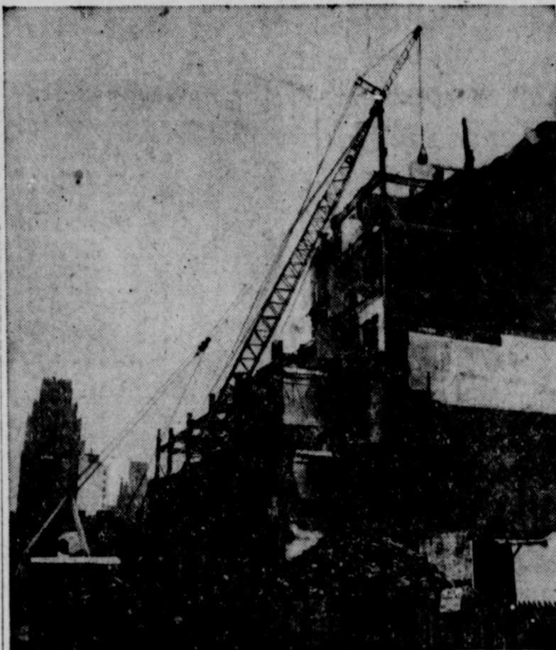
DESTRUCTIVE BALL GAME . . . The engineer at the controls of this giant crane has to keep his eye on the ball, literally. The pellet he is swinging, a two-ton steel sphere suspended from a 120-foot boom, is being used to demolish a building in the vicinity of New York's East river where a site is being cleared for construction of the United Nations world capital.
