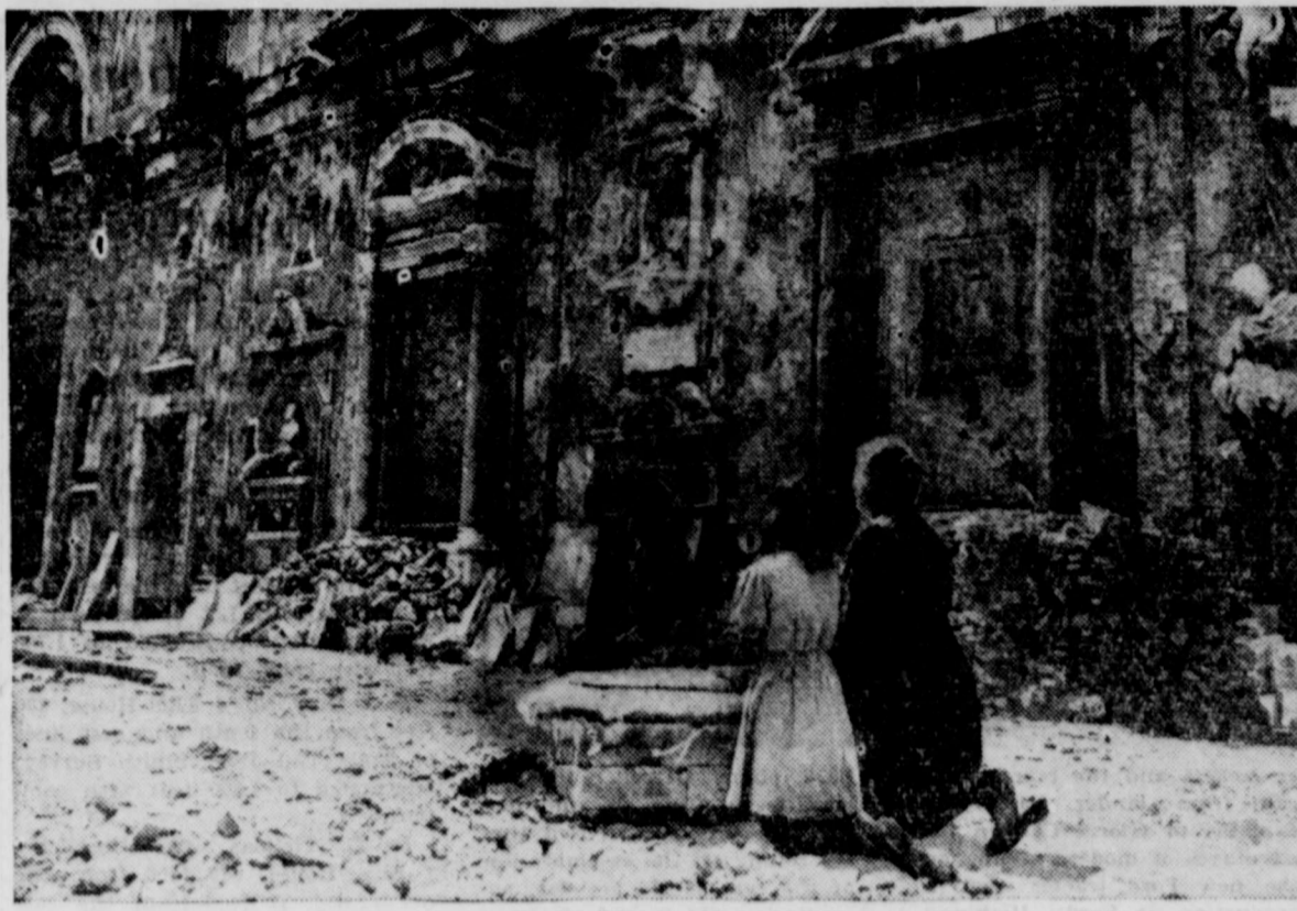
FAITH IS INDESTRUCTIBLE . . . The beautiful cathedral at Liphorn, Italy, ravaged by the war, is now little more than the spirit of a place of worship. Some of the debris has been cleared up, and all that was salvageable was saved for use in reconstruction. Meanwhile, the people continue to go to the ruins to pray as they always did, for neither bombs nor shells nor the destruction of their cathedral could dent their faith.
