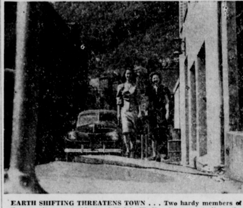
EARTH SHIFTING THREATENS TOWN . . . Two hardy members of the opposite sex, residents of Welch, W. Va., brave a stroll on the buckled streets of the town after sections of the little city started to sag alarmingly because of a mysterious shifting of the earth. Huge cracks appeared in several large buildings, and inhabitants were fearful that their homes would be destroyed.
