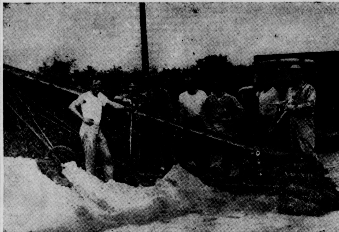
'KNOW-HOW' HELPS DEFEAT FLOOD MENACE . . . With the Mississippi off on one of its most destructive henders in a century, farmers up and down the river were hard put to keep the rampaging waters from flooding their fields. At Wapello, Ia., this crew of flood fighters rigged up a portable grain elevator to carry sandbags up to levee in background for speedier reinforcement and to eliminate necessity of workers' hauling heavy bags up the slippery 12-foot embankment.
