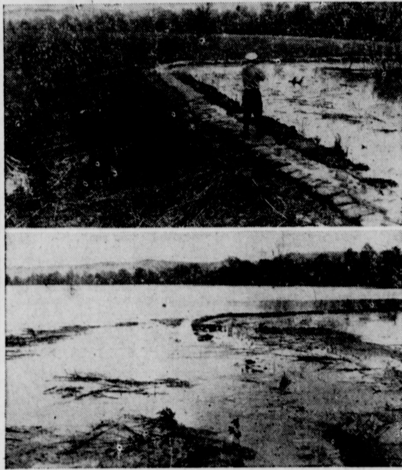
'BIG MUDDY' RUNS AMOK . . . Abnormal spring rains are causing floods in many parts of the country, inundating large tracts of land. Top panel shows the sandbagged levee of the Missouri river near Aldridge, Ill., before the rains came. Below, 36 hours later, the levee proves no barrier, the water breaking through to flood 2,000 acres of farm land.
