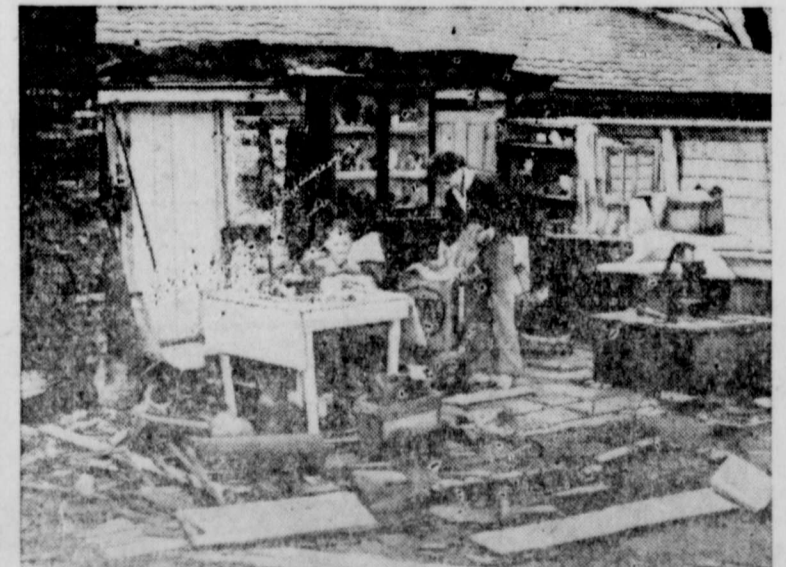
MAN, NOT ELEMENTS, CAUSED THIS . . . It looks as if a cyclone had struck the Jim Munro home at Le Claire, Iowa. However, it was the landlord, not the elements, that caused this scene, the Munro family claims. They charge the landlord, Harold Olsen of Montpelier, Iowa, wrecked the summer kitchen of their home when they ignored an eviction notice. Similar happenings have been reported in other parts of the country by landlords anxious to gain possession of homes.
