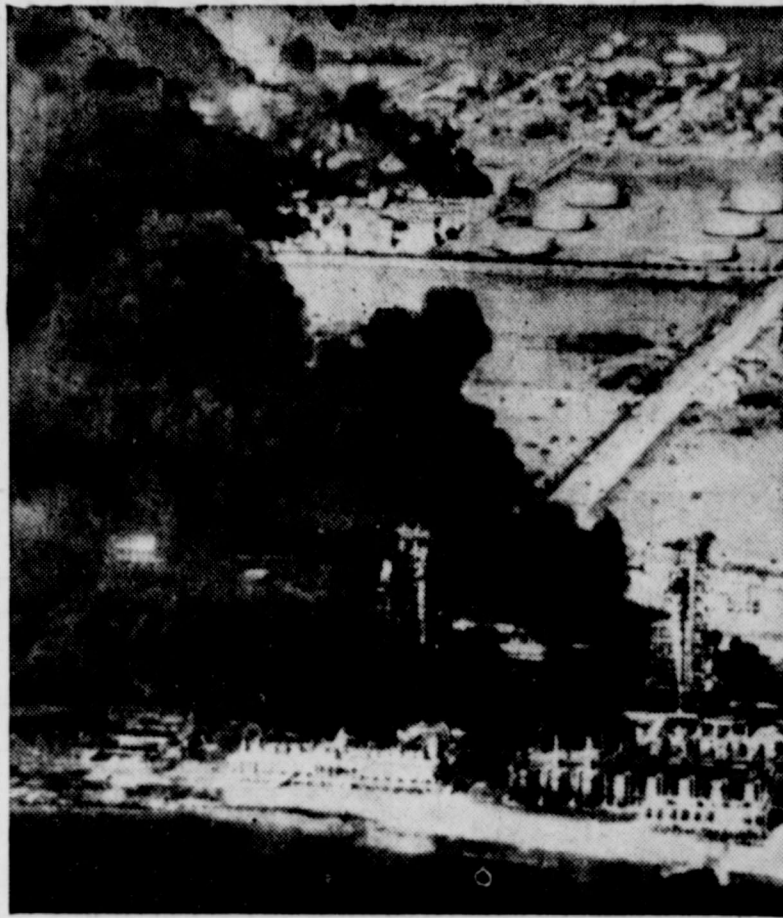
AS TEXAS CITY STARTED TO BURN . . . Closeup airview of the burning Monsanto works and oil dumps when the flames began creeping up to the oil depots at Texas City, Tex., during the early stages of the explosion and fire. Damage within the confines of this photograph were estimated at more than $35,000,000. Explosion at the Monsanto works ignited a pipeline which exploded, causing the oil dumps to catch fire during the early hours of the disaster.
