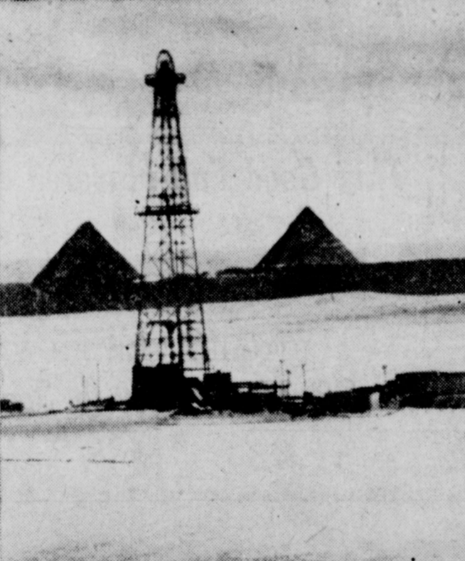
OIL IN SHADOW OF PYRAMIDS . . . Abu Roash well, drilled by Standard Oil company, is shown with the famed pyramids of Giza forming a background. This well, begun in January, is a wildcat one, drilled to determine if the desert can contribute a share of oil to the mechanized world. Other wildcat wells are planned by the company. When photo had been taken the drill bit had chewed down 5,100 feet into the land of the Pharaohs.
