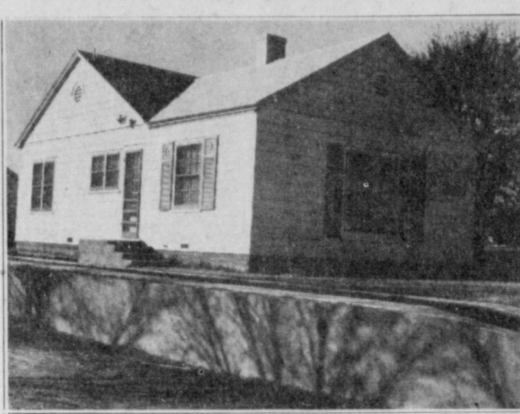
Presented in this picture is the modernistic four-room frame home of Mr. and Mrs. Gaither Bell, located at 1910 29th Street. Hardwood floors are utilized throughout in the structure, which has a kitchen-breakfast room, two bedrooms, living room, bath and hall.
