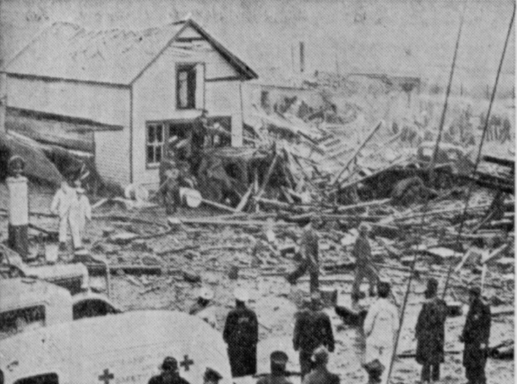
WOODBRIDGE, N. J.—This scene of desolation met the eye after a terrifying blast leveled the United Railway and Signal Co., here, killing nine persons and injuring 33. Though the plant made torpedo signals for railroads, it was said to be working on a device of "great importance" to the army and navy.
