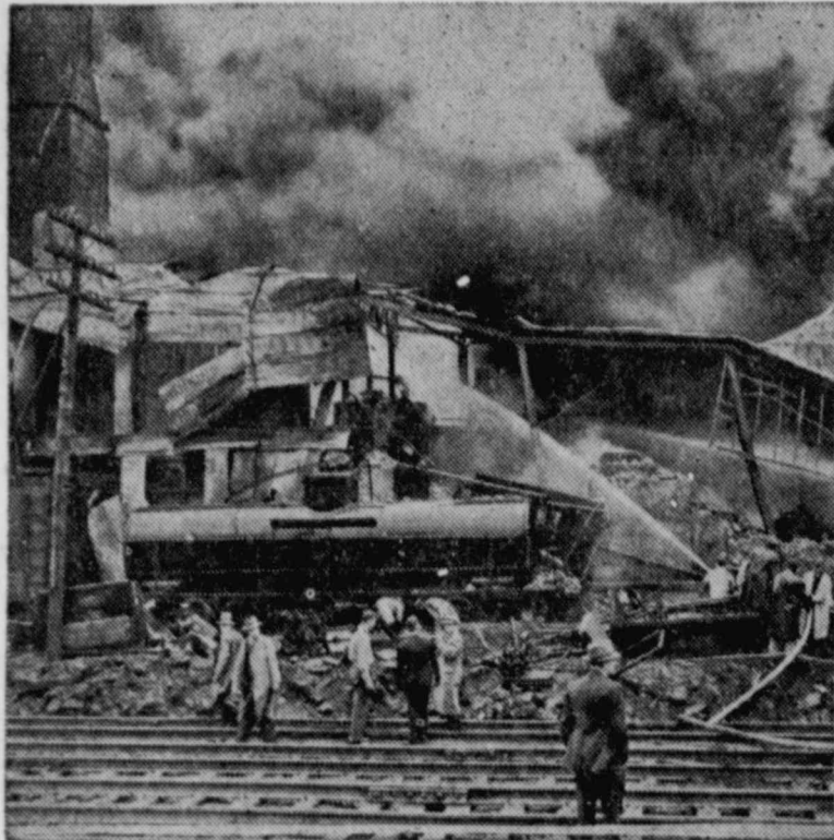
The burning ruins of two buildings are shown in the above photo of the Pennsylvania Industrial Chemical corporation at Clairton, Pa., which was damaged by an explosion of resin and oils. The blast resulted from "adverse chemical reaction" in an agitator. Six persons were injured in the blast. The damage is estimated at $50,000. Flames were brought under control an hour after the explosion.
