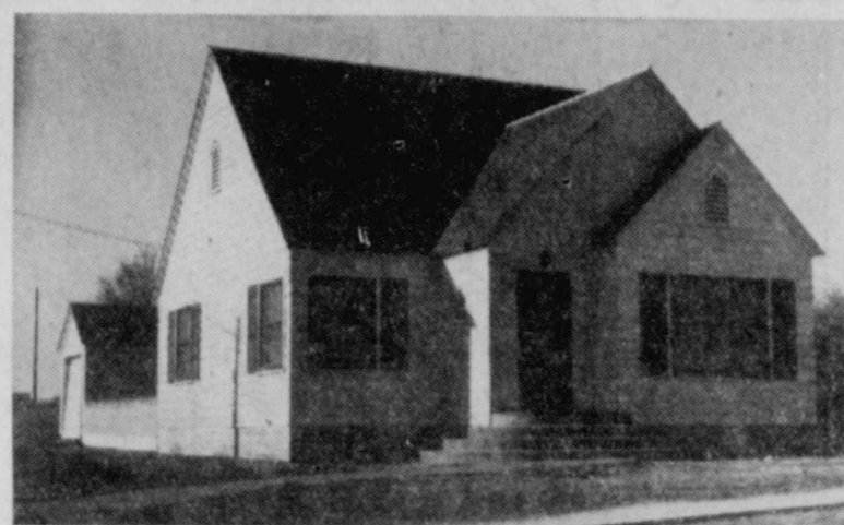
Shown this week is the five-room frame structure, with bath, that has been erected by R. J. Randalls at the corner of Avenue S and 30th Street. Another modern home for Snyder,
