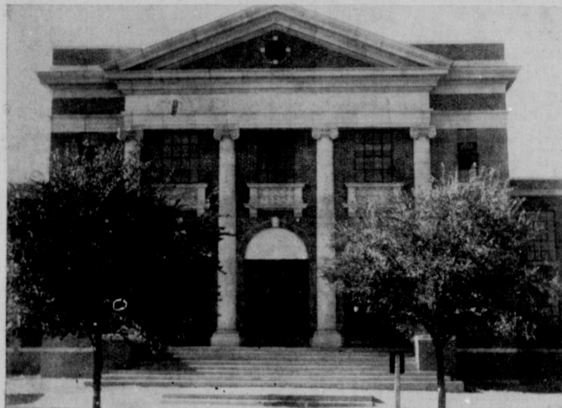
This view from the north side of Snyder's new $145,000 school plant gives an excellent view of
