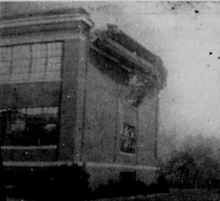
In this action shot of Snyder's most destructive school fire last year, a part of the northeast wall is being pulled down. Notice the giant mass of brick, concrete and steel was just leaving its flame-enveloped mooring as High School Student Bill Miles' tiny camera clicked. Center of the building is smoldering here.
