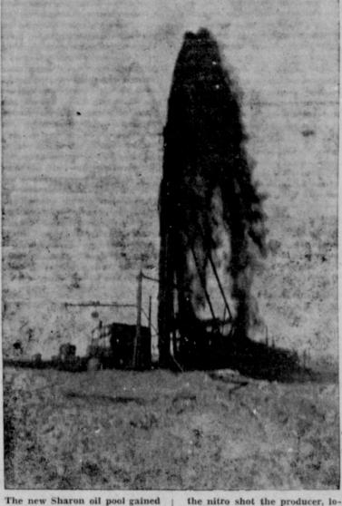
the attention of Central West Texas oil operators when the Coffield & Guthrie No. 1-A 4st National Bank 3185-foot test, shown above, was shot recently with 580 quarts of nitro in upper pay saturated sections from 2,232 to 2,412 feet. Following
