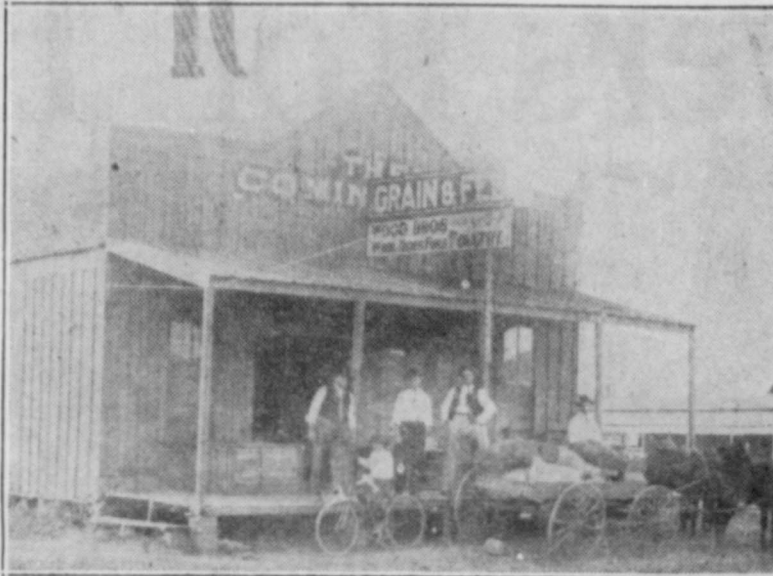
"The Coming West," Scurry County's first newspaper, was housed in this frame structure
