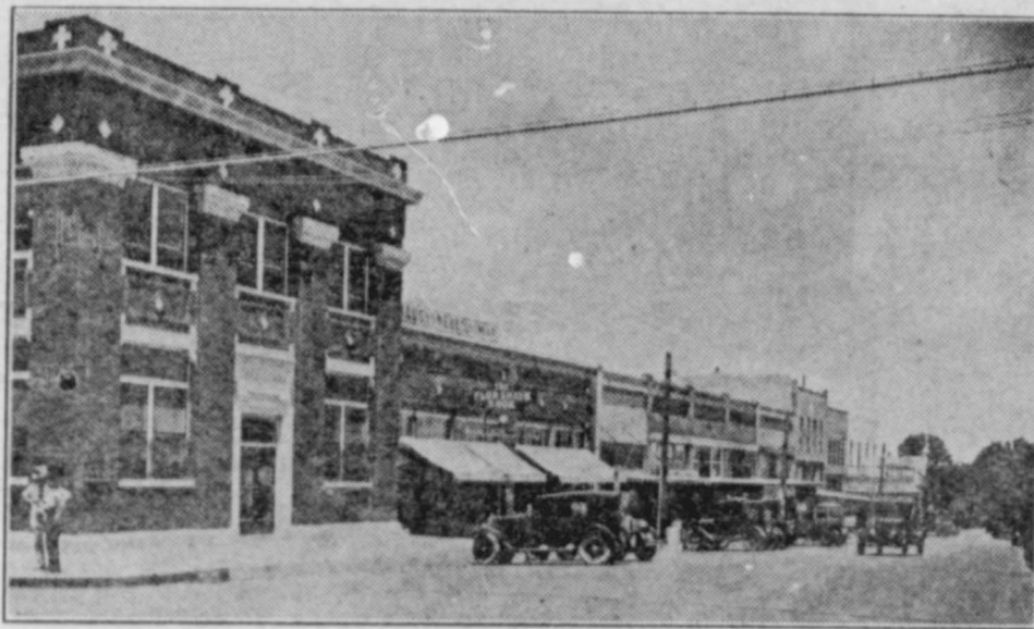
This substantial banking house on the northwest corner of the public square is the home of Snyder's and Scurry County's only
