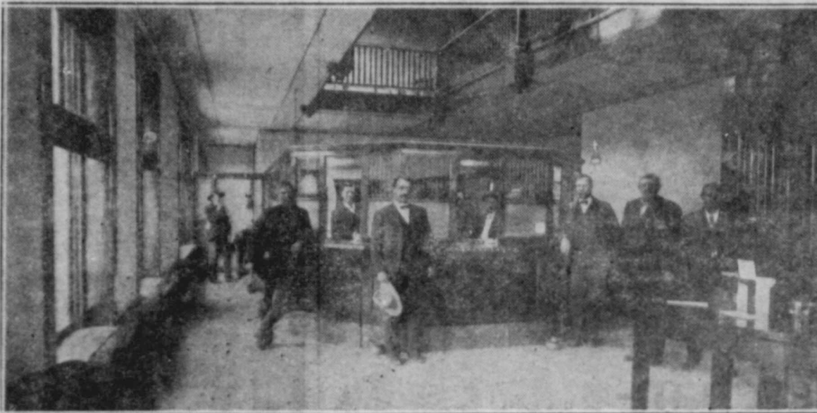
This picture of the old First National Bank, taken in 1916, reveals several of Snyder's old-timers. The institution stood on the northwest corner of the square, now the H. G. Towle Jewelry Company site. The first two men on the left are un-
