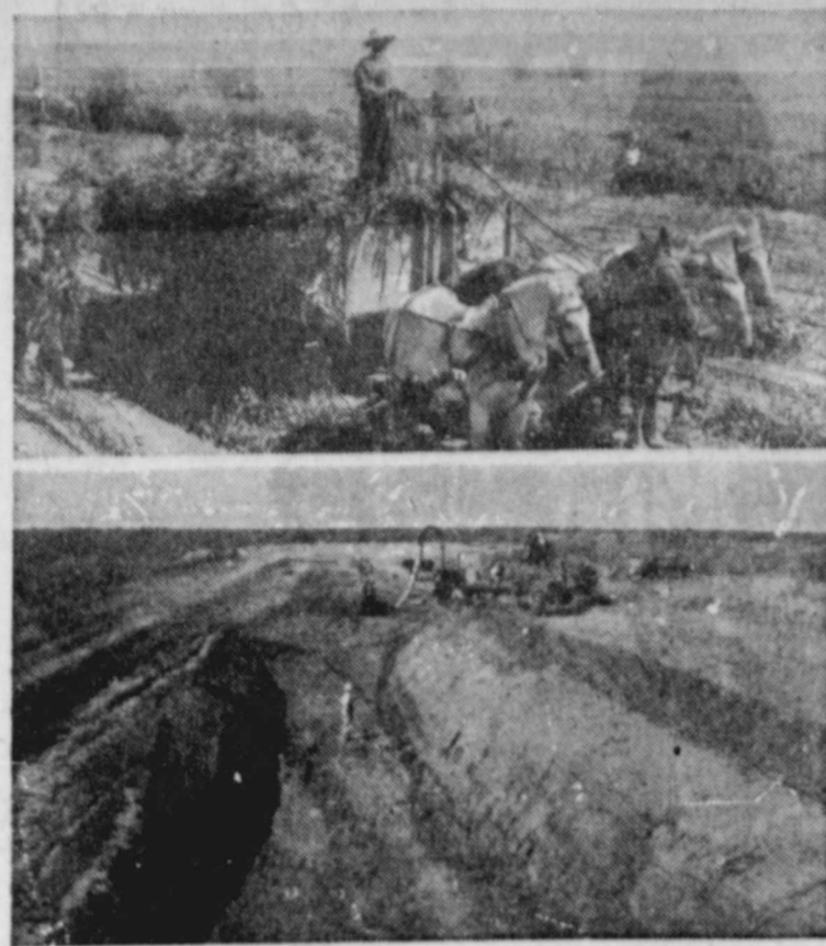
Dallam County's largest trench silo, an 800 ton affair on the Cecil C. Jones place near Texline, is pictured here. Jones, who in 1923 worked with the county agricultural agent and the Extension Service division of Texas A. & M. College to put in the first trench silo in his section, a
