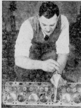
Measuring cylinder went with a precision gauge—accurate to a hundred-thousandth of an inch!
