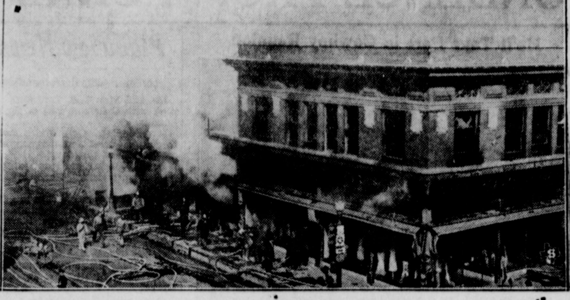
More than $300,000 damages was done when this quarter of a block of downtown El Paso was destroyed by fire, and 14 firemen were injured fighting the blaze. It took nine hours to completely subdue the flames. Police and fire authorities are investigating, believing the fire might have been of incendiary origin. A clothing store, photo shop, jewelry and paint stores and many offices went up in smoke.
