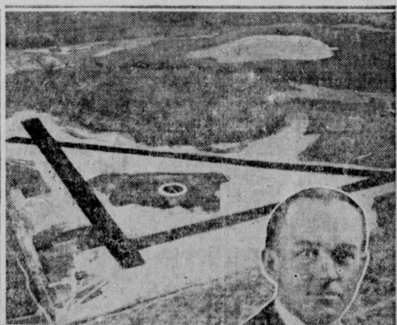
Birds-eye-view of Municipal Airport, Jacksonville, Fla., with asphalt paved landing strips.
