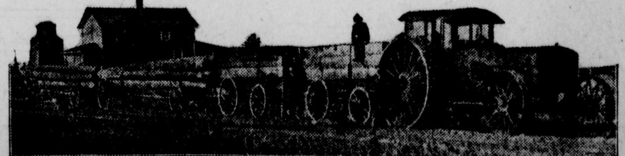
This Method of Hauling and Grading Is Said to Save 50 Per Cent Over the Old Method.
