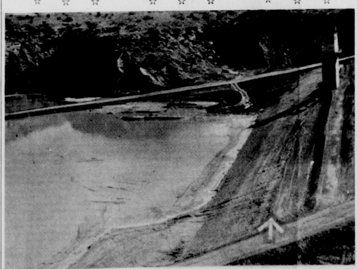
This picture of the Mackenzie dam shows the tower-like structure which is the draw-down or feeder line for the filtering plant. The water line (indicated by arrow) shows where about 25 feet of water was backed by the dam from earlier rains. This put the construction company's road, etc. underwater, and they had to let most of the water out. Water is being released through the draw-down all the time now.
