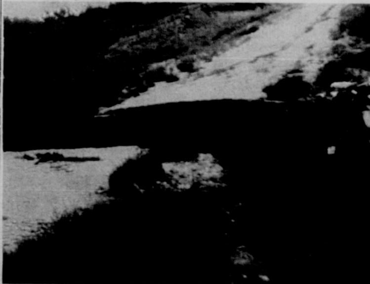
Rainfall has been heavy in parts of Briscoe County during the past week. In the area along the Caprock, rainfall totals have been upward of five inches in places, putting water over the spillways of some of the county's lakes and washing out some earth dams. One dam broke sending down a wall of water that washed out a bridge west of Quitaque on the farm road that leads to Cottonwood Lake. Silvertown rainfall has totaled 1.42 inches since last week.
