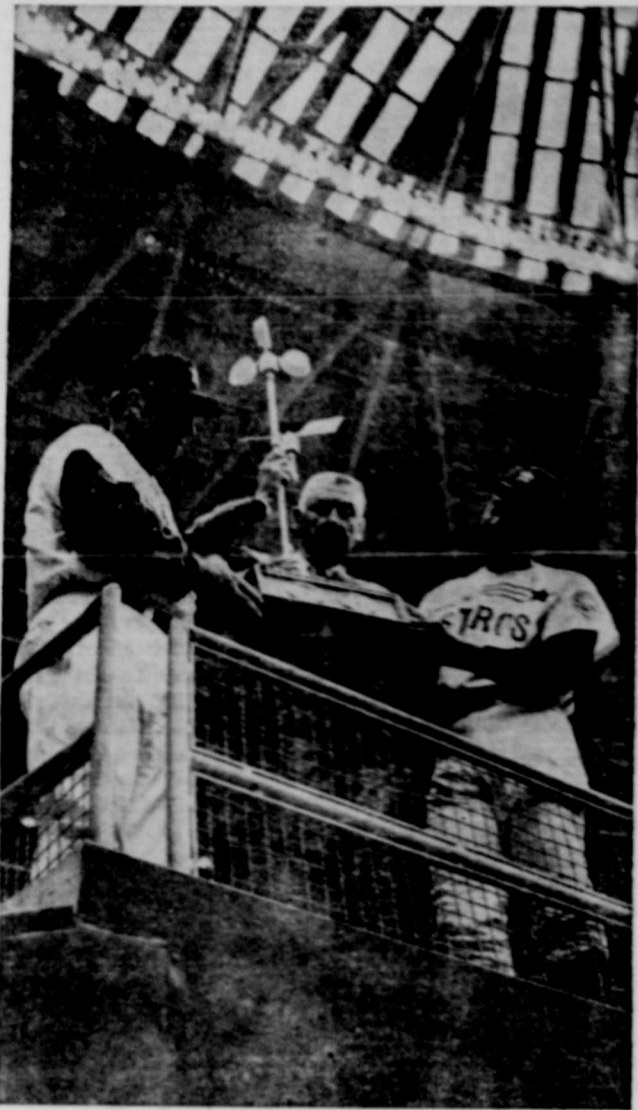
ASTROWIND OR NO ASTROWIND? Investigating reports that the Houston Astrodome's air conditioning system may be partly responsible for a doubling of home run production there this season, Charles Kaufman, a Carrier Air Conditioning Co. engineer, checks air movement with an anemometer. Fred Gladding, left, top Astro relief pitcher, and Jay Alou, one of the Astros' leading hitters, protect their respective interests in the outcome. The verdict by Kaufman—no wind, just muscle.
