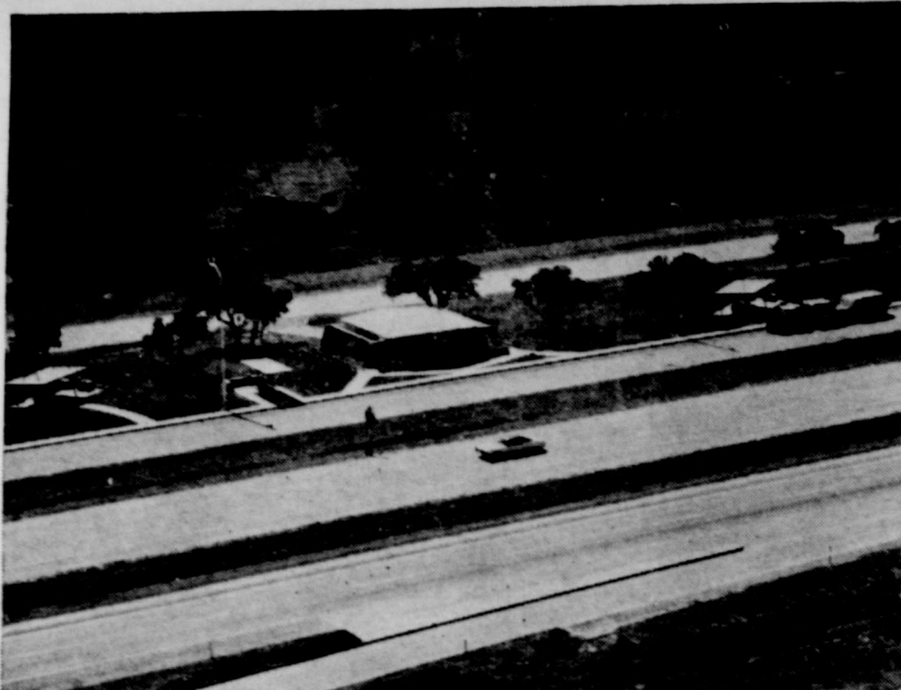
Situated just off the main lanes of Interstate Highway 35 near Georgetown is this Texas safety rest area complete with rest room facilities, picnic shelters, grills, trash disposal, drinking water and a travel information display. For the benefit of motorists the Texas Highway Department supplies all the comforts of home.--TEXAS HIGHWAY DEPARTMENT PHOTO.
