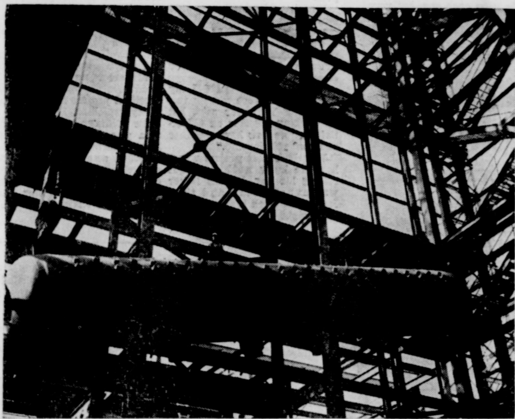
Continued construction on a 210,000 kilowatt generator at Nichols Station, northeast of Amarillo, is part of Southwestern Public Service Company's $20,000,000 improvement program for 1967. Pictured is the installation of a 225,000 pound boiler drum for the new generating unit.
