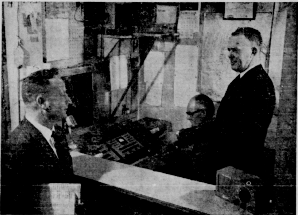
COMMUNICATIONS CENTER at Wadesboro, N. C., combines a round-the-clock civil defense nerve center with a unified radio service for local police, fire and sheriff's departments. Used for this dual purpose, the equipment is kept in top notch condition at all times to meet emergencies. At the radio is Waldo J. Stroud, one of three operators hired by the local CD unit under a program in which Federal and local governments share the costs of new civil defense employees. Raymond H. Northcutt (right), Wadesboro-Anson County CD director, explains his radio setup to Herman J. Sisk, Area E director for the North Carolina Civil Defense Agency and one of five area directors hired under the same cost-sharing law to help build up CD at the local level. (OCDM Photo)
