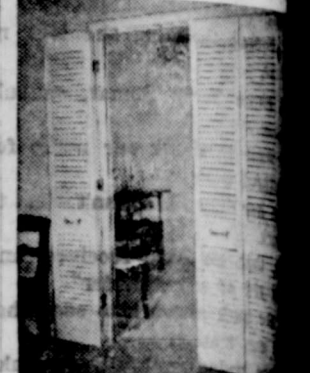
Louvers with special hardware fold to the sides when door is closed.
