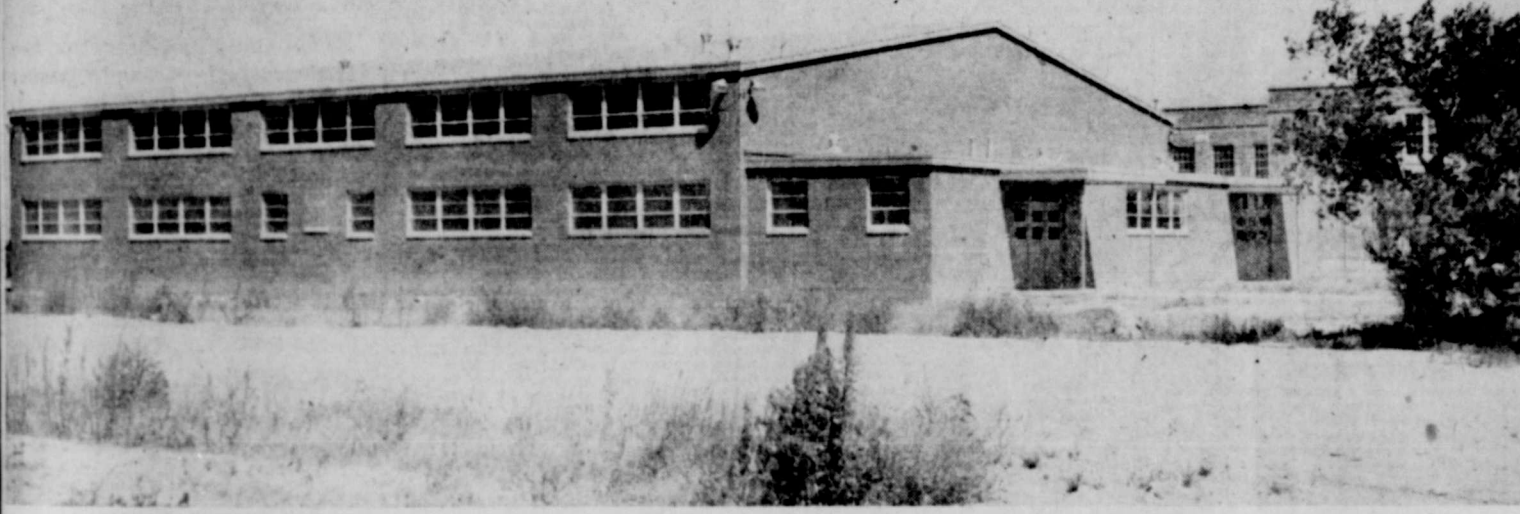
NEW GYMNASIUM READY FOR USE—Pictured here is Silvertton's newly completed modern gymnasium which has been recently completed and accepted by the school board. The floor space consists of 12,000 feet. Has seating capacity for 840 people. It also has a full size court which will enable the school to take care of any indoor sports. It also has four dressing rooms fully equipped with showers, etc.
