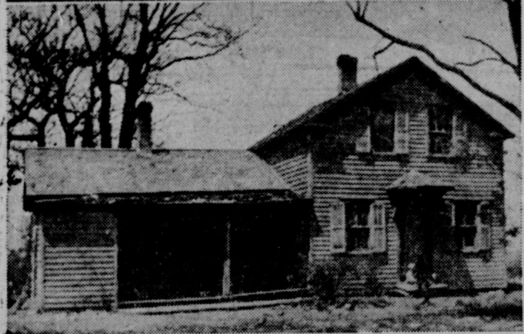
The handsome, new-looking home, top, is the remodeled version of the 100-year-old farmhouse, bottom. Window rearrangement, elimination of the porch, a new fire-resistant asphalt shingle roof, and new paint were principal exterior improvements.
