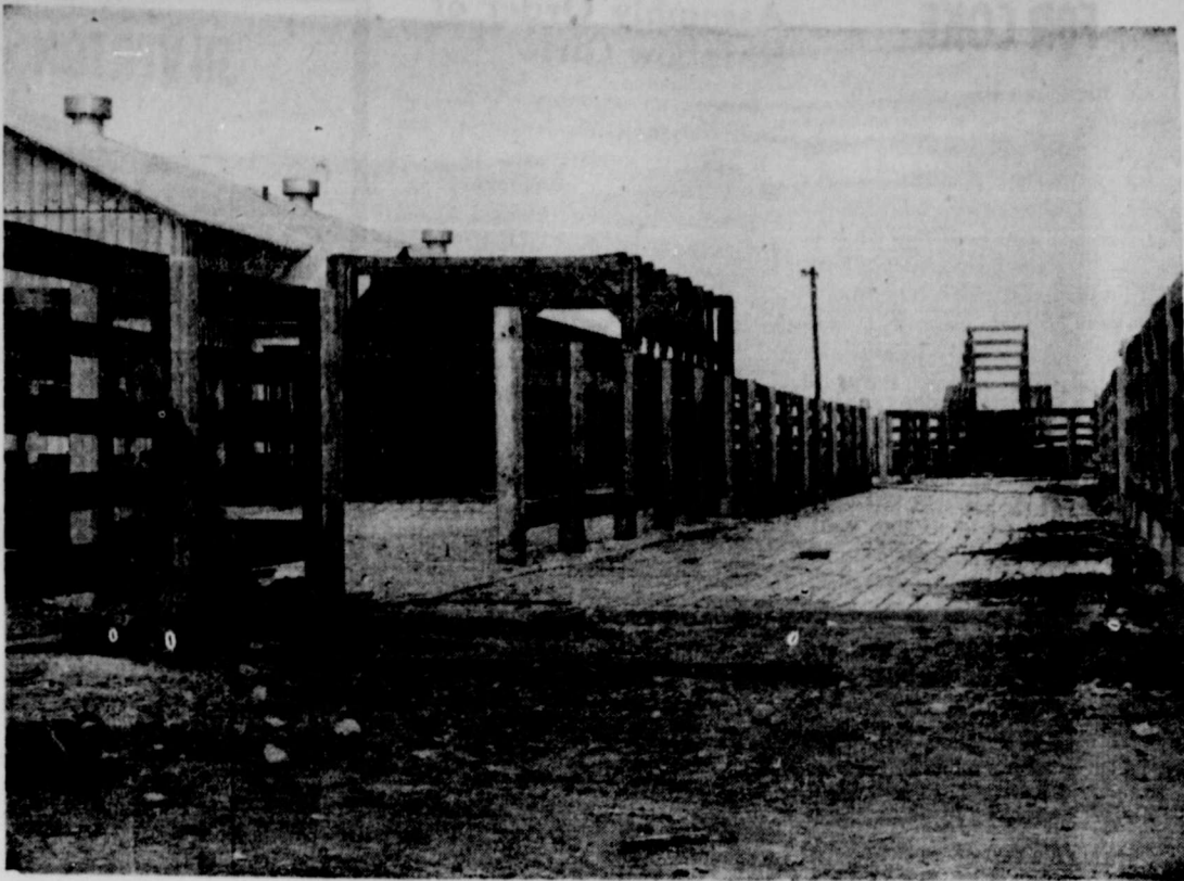
View of the partially completed loading docks and pens at the new Amarillo Stockyard. This photograph shows the concrete post and oak panel construction of the pens and the incomplete hard surface that is to be installed in approximately half the pens. Also shown at the left of the picture is the rear of one of the administration buildings and the Fairbanks-Morse Scale that will be used to receive cattle at the yard.
