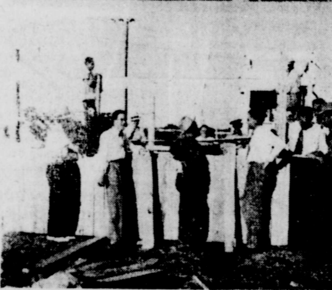
The new rodeo arena and grandstand recently built in Plainview will be the scene of the Plainview Frontier Days rodeo to be held July 17-18-19. Citizens of Plainview who volunteered their labor three nights in order that the stands might be completed more quickly are shown above as they worked. The rodeo stock is to be furnished by Buck Steiner & Sons of Austin.
