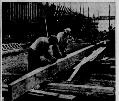
Two shipwrights work on a keel here. In the background are two hulls in various stages of construction.
