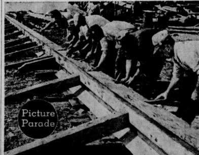
Greasing the skids before launching a completed wooden ship. Pounds and pounds of grease are smeared on the skid to make the slide of the new craft easy and to counteract friction.
