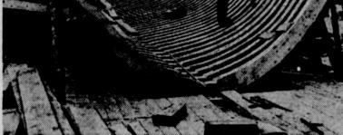
Old-timer Ray Rubshaw is working inside the framework of a hull under construction. He is dubbing or smoothing out and lining up the ribs for planking, using an adz.
