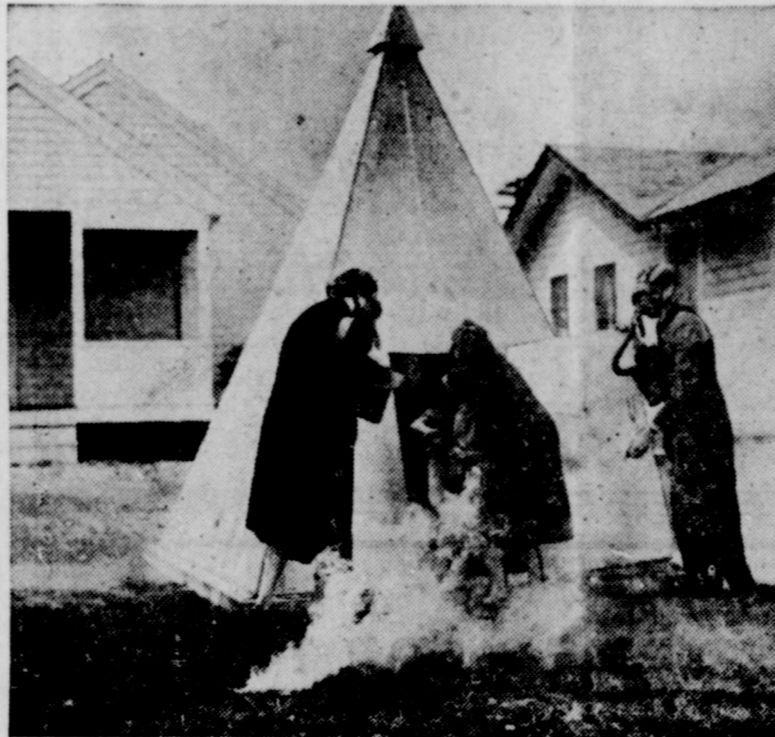
Mass production air raid shelter, shown during a tryout in Boston. It is bolted on a concrete base. Ventilation comes in at the top where the little cone crowns the steel pyramid. Yes, this shelter can accommodate 12 people. With air raid alerts on both coasts, interest in shelters is increasing. Some can be bought for as little as $200.
