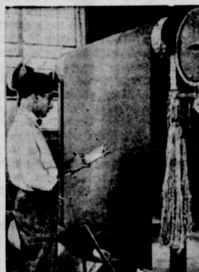
Trained eyes scan every inch of this bolt of cloth as it is unwound from roller to roller. A defect would cause rejection.
