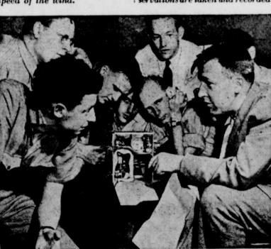
Professor A. Spilhaus explains the operation of a radiometeor ograph to some of the student weathermen. Attached to a balloon, it is sent aloft to ascertain conditions in the upper air.
