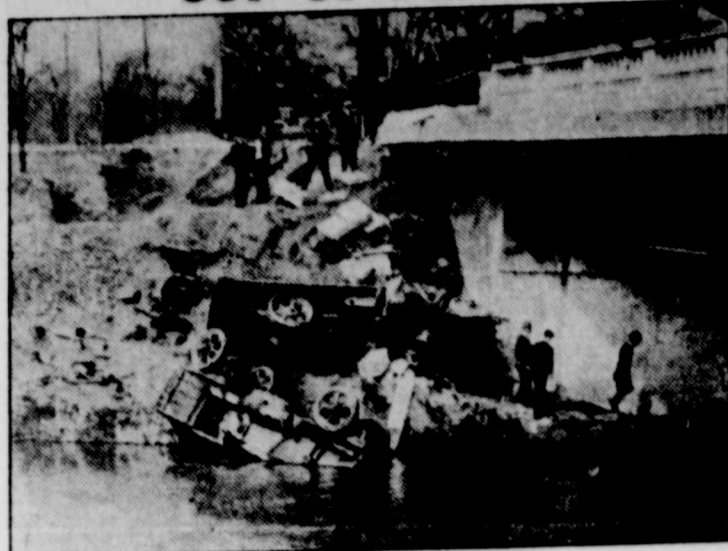
The above scene shows the finale of a crash between two trucks, hurtling through a concrete bridge approach with a crushing impact as if a piece of frosting were flicked from a birthday cake.
