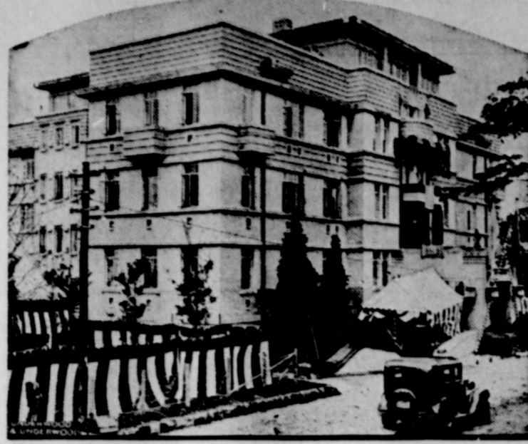
The first Rockefeller foundation contribution to the cause of Japanese education is this new building which forms part of the greatest private university of Japan, the Keio university. The building is constructed of double reinforced concrete and represents the new type of earthquake-proof architecture.
