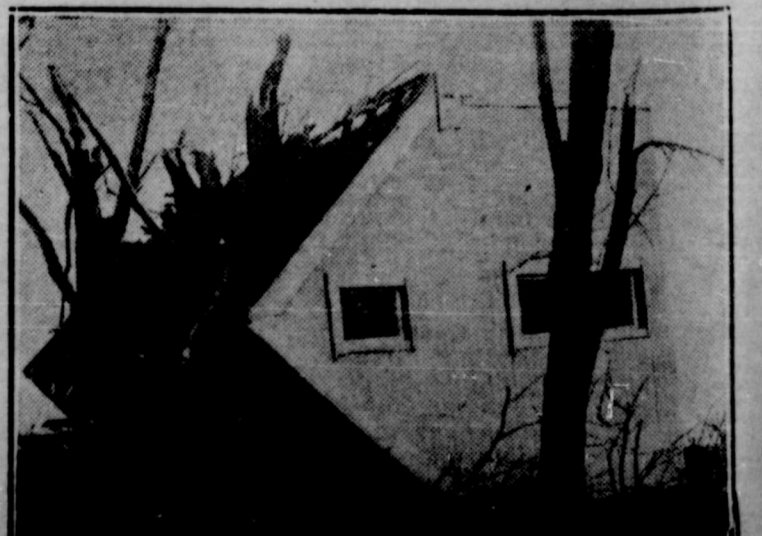
The storm played strange pranks. Here is a house turned on its side and lodged between two trees on the Main street of Griffin. The glass windows were not broken.
