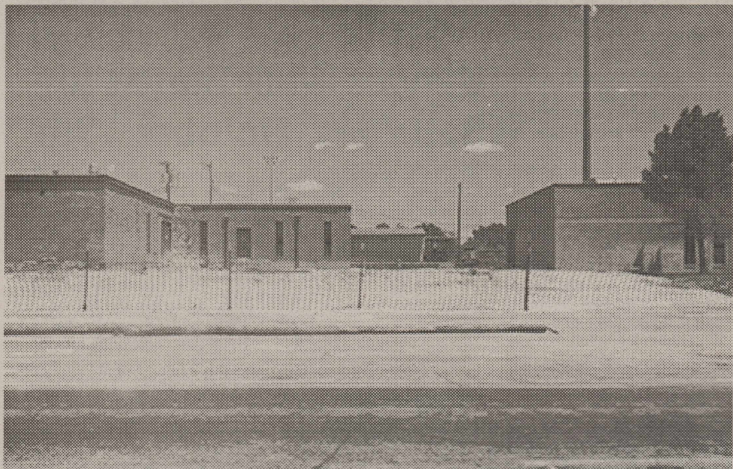
Ready for the New Band Hall - The construction zone between the junior high and high school is blocked off ready for the building of the new band hall. Exercise caution in the area.
