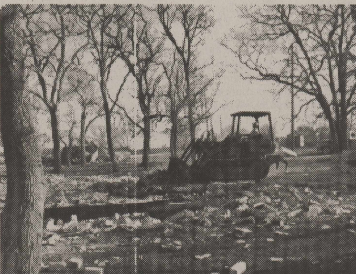
The massive cleanup after the fire.
