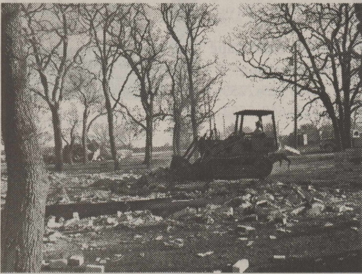
The massive cleanup after the fire.
