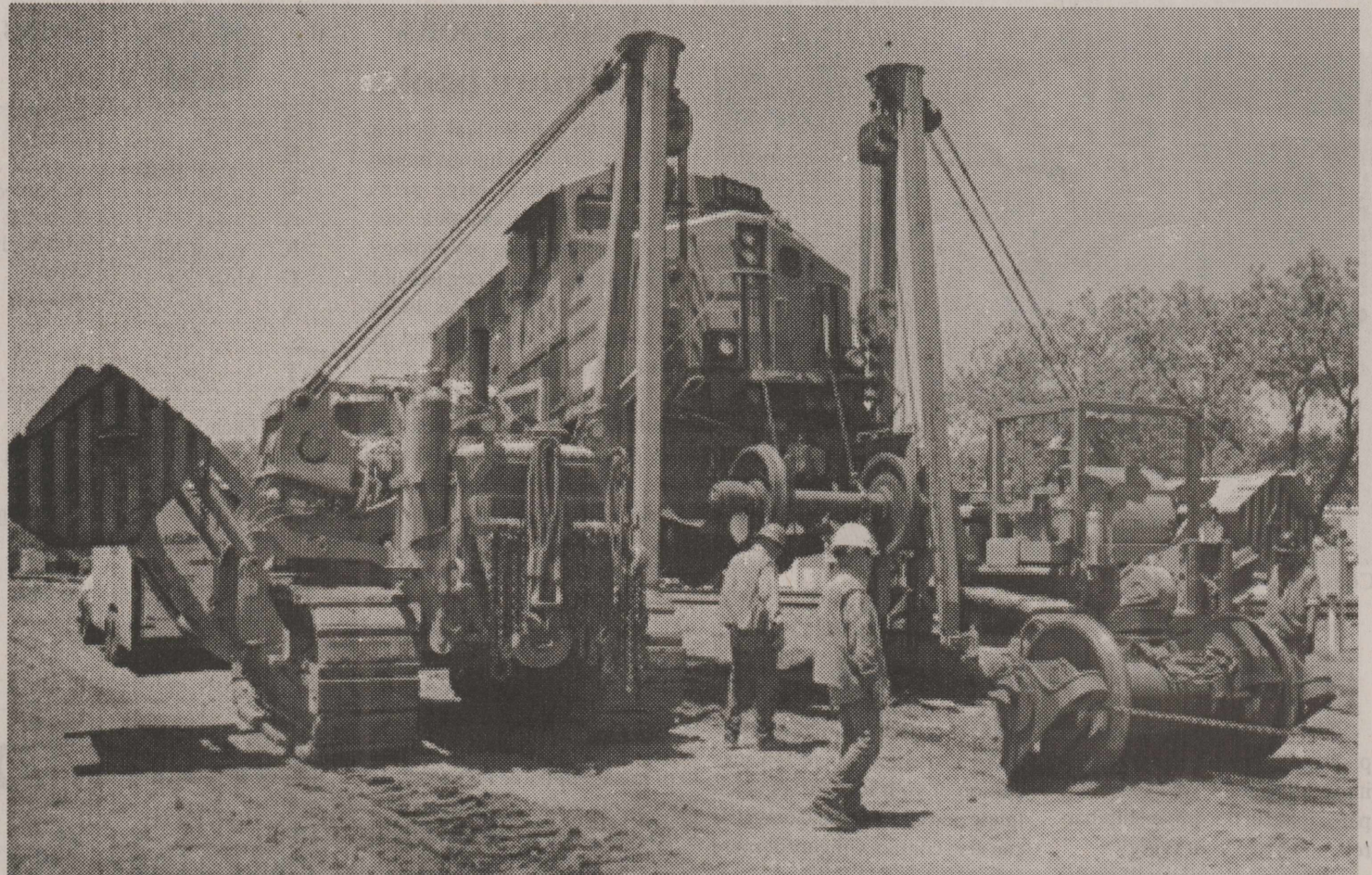
REPLACING A TRAIN ENGINE WHEEL —A construction crew from JR's Crane & Excavation Inc. from Greenville, Texas lifts a 400,000 pound train engine on the Union Pacific train track sidetrack north of the Dollar General store in downtown Clyde on Thursday, May 8th to replace a train engine wheel which had locked up earlier in the week. The train pulling the railcars sat idle in Clyde for two days until the crew was able to remove the train engine. The train engine wheel was replaced and gone by Saturday, May 10th.
