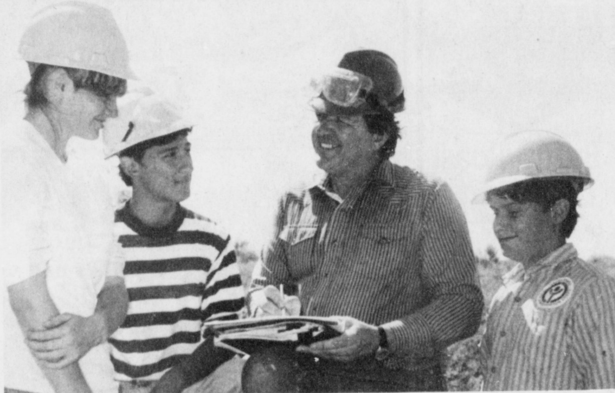
YCC WORKERS--at the Muleshoe National Wildlife plan a better way to build a new footbridge. They are (left to right): Stephanie Gore of Sudan, Michael Mendoza of Muleshoe, Tom Boutell, YCC Director, and Alan Black of Sudan. (Journal Photo)
