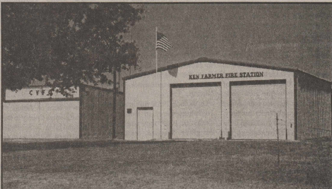
COTTONWOOD'S NEW FIREHOUSE — The Ken Farmer Fire Station, dedicated to the memory of Cottonwood Fireman, Ken Farmer, who died suddenly in May 2009. Farmer spearheaded the fund-raising campaign and the construction of the building. At left, is the old Cottonwood Firehouse erected in 1988. Volunteers repainted the building for the dedication ceremony.
